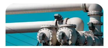
For 2023, we have planned the modernization of water pumping systems used for sanitation services and the supply of soft water to textile machinery. Installing speed variators in the water pumps and maintaining constant pressure in the water pipes will help reduce current spikes during pump starts, and electricity consumption will be adjusted according to demand in the plant. This transition will result in a 30% reduction in electricity consumption compared to the old system.
